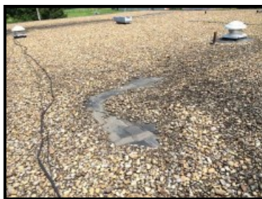
Past repair attempts to the roof system can be seen here.
